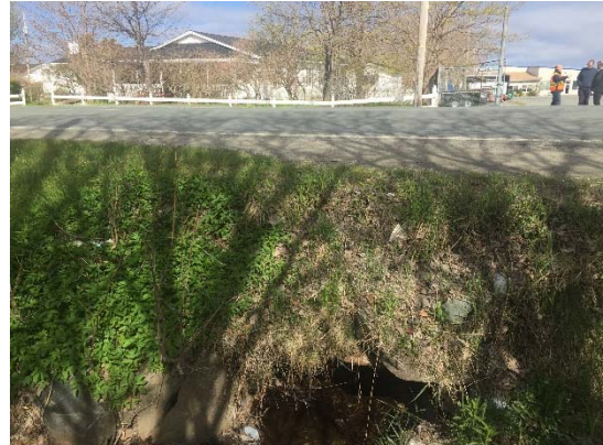
Figure 8: 1200mm CSP Culvert Heading towards Cronin's Place Property
