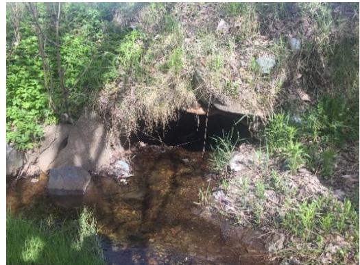
Figure 7: Runoff Stream Leaving Culvert Crossing Peacekeepers Way
