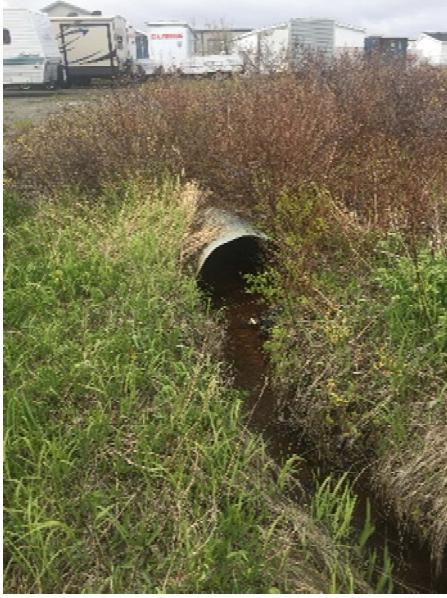
Figure 3: 900mm CSP Outfall - Country Trailer Sales Ltd.
