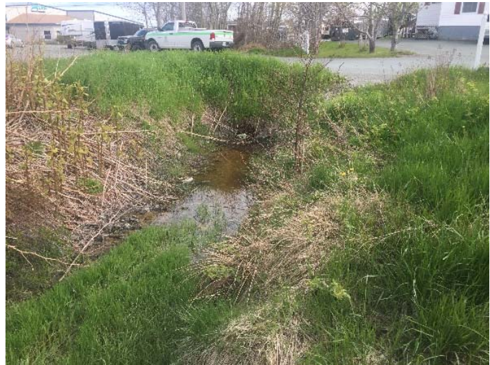
Figure 4: 600mm CSP Culvert - Cronin's Place
