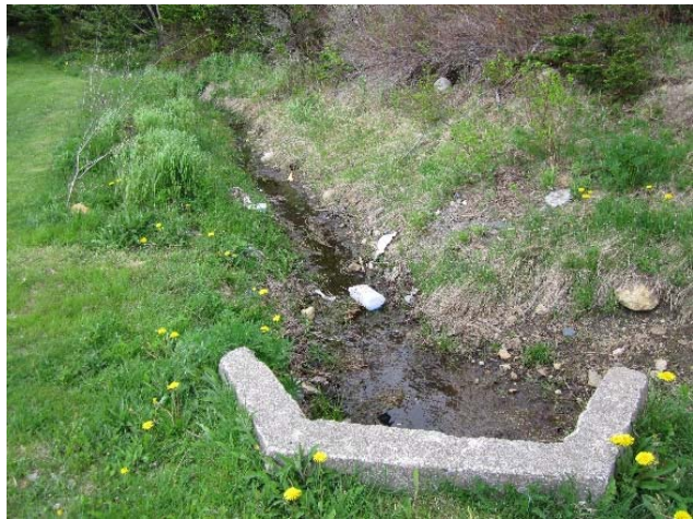
Figure 2: Headwall - Cut-off Ditch - Jerathon Place
